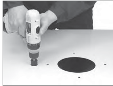
(6) Cut hole for oil return tube (if required).
