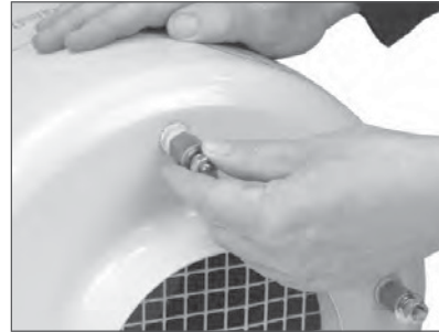
(2) Fit 4 x case studs (supplied with unit).
